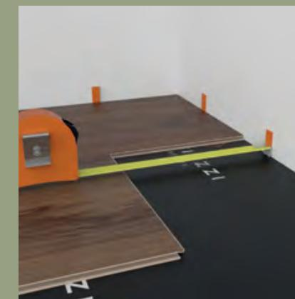
**Step 4:** At the end of the first row, put a spacer 3/8" (9,525mm) to the wall and measure the length of the last plank to fit.
