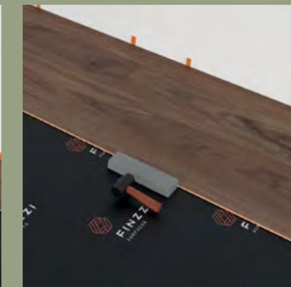
**Step 9:** After 2-3 rows. Adjust the distance to the front wall by placing spacers 3/8" (9,525mm) on the side walls and the end wall. Once the adjustment is done against the main wall, continue to install till the last row.
