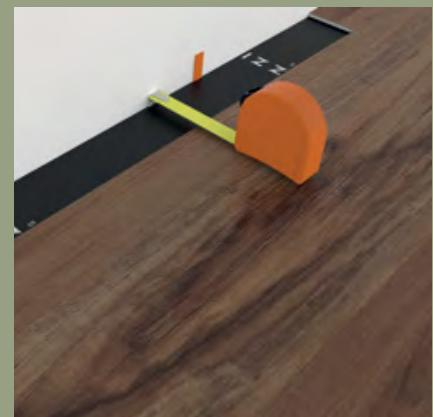
**Step 10:** Last row. The Minimum width of the last plank should be NOT LESS than 2" (5mm) wide. Put a spacer before measuring. Cut the panels lengthwise and glue the short ends.
