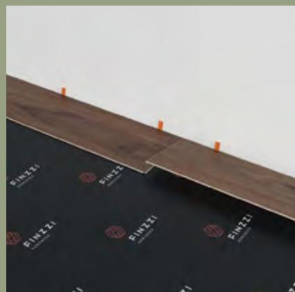
**Step 3:** Fold the panel down in a single action movement. Afterwards press down or slightly tap down at the short end just installed till it clicks.
