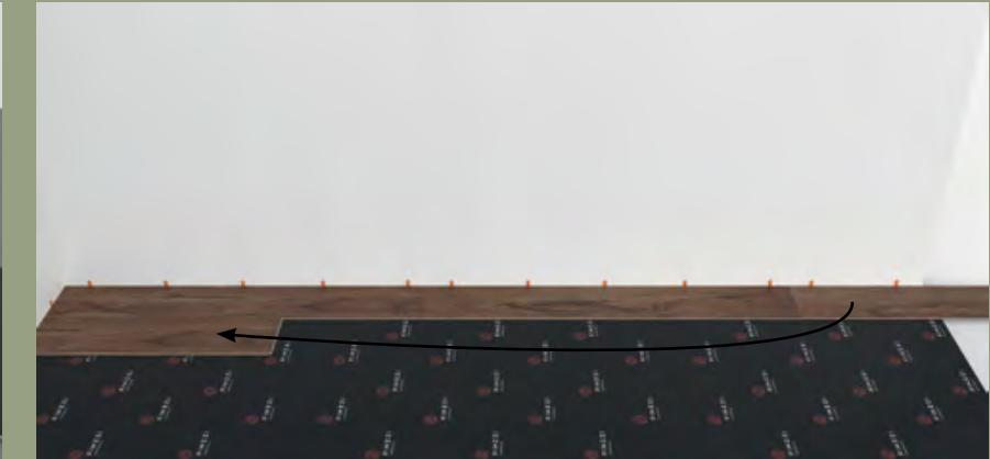
**Step 6:** Starting the second row the first plank should be a min length of 10" (254mm). Put a 3/8 (9,525mm) spacer against the wall and measure the last piece. If it is shorter than 10" (254mm) a new starter piece should be used. Insert at an angle into the previous row and tap (on the long side) it in using a tapping block till flat.
