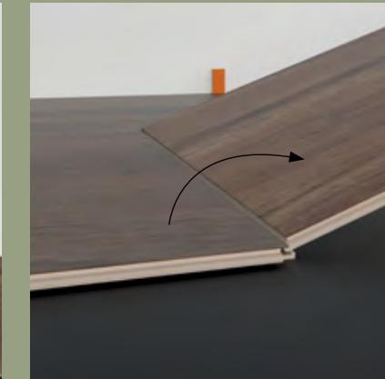
**Step 8a:** Second plank, second row. Place the panel at an angle into the groove of the previous row making sure that the end of the panel is tight/flush to the short end of the previous panel.
