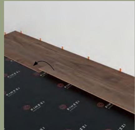
**Step 8b:** Fold the panel down in a single action movement with a slight press to the left to the short end of the previous panel. Again, using the tapping block tap it against the long end into the previous row.
