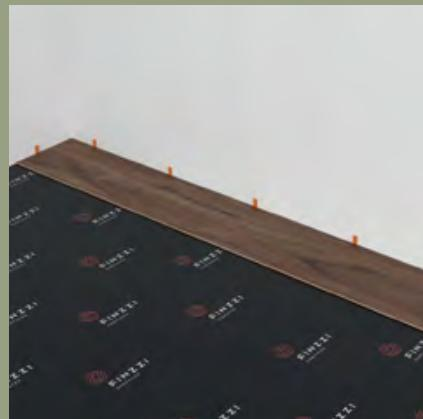
**Step 1:** First plank, first row. Place a spacer of 3/8" (9,525mm) thickness to the left and position the plank against the wall.
